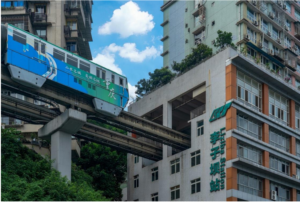
Figure 1 Chongqing Rail Transit line 2 scenic spots Liziba Station using light rail monorail system.
